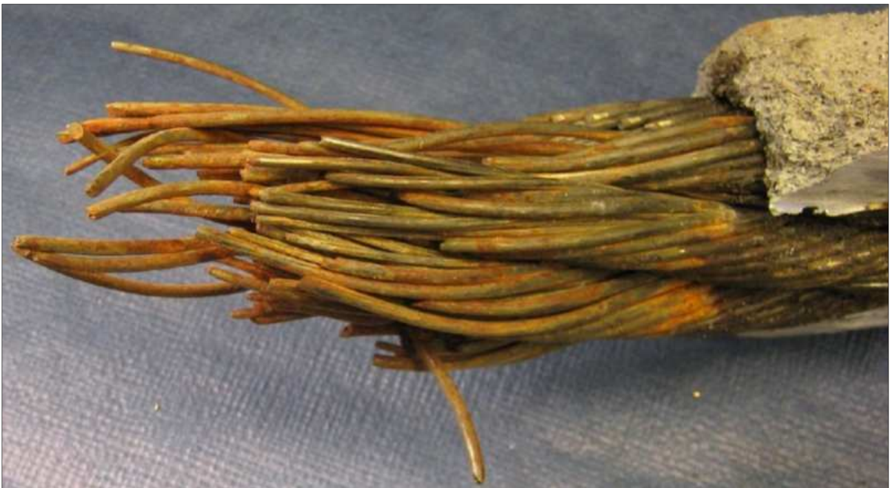
Figure 10: Close-up of the wire fracture Source: FORCE Technology
