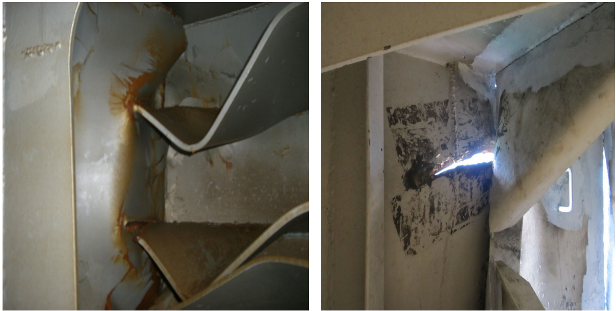
Figure 10: Damage to the bow of ANKARA (2)
