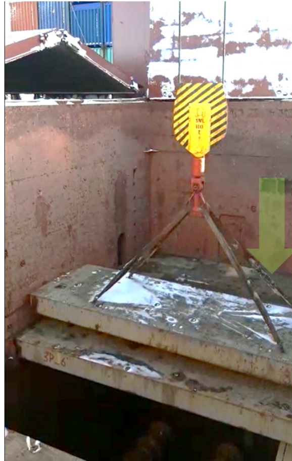
Figure 4 - Pontoon N°5 lifted
