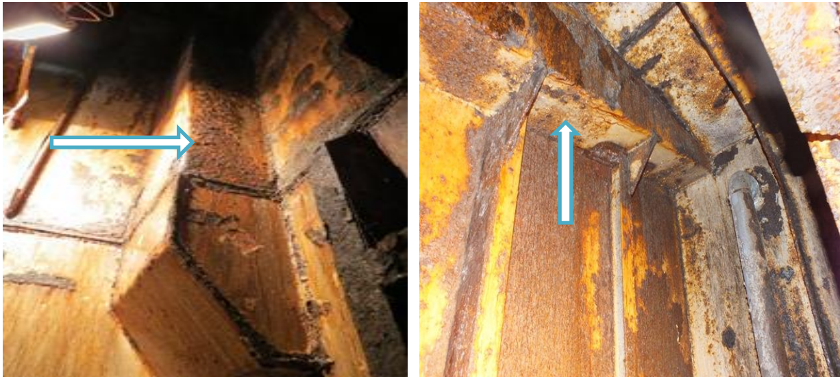
Photograph 7. Air conditioning ventilation trunk before the repair.
