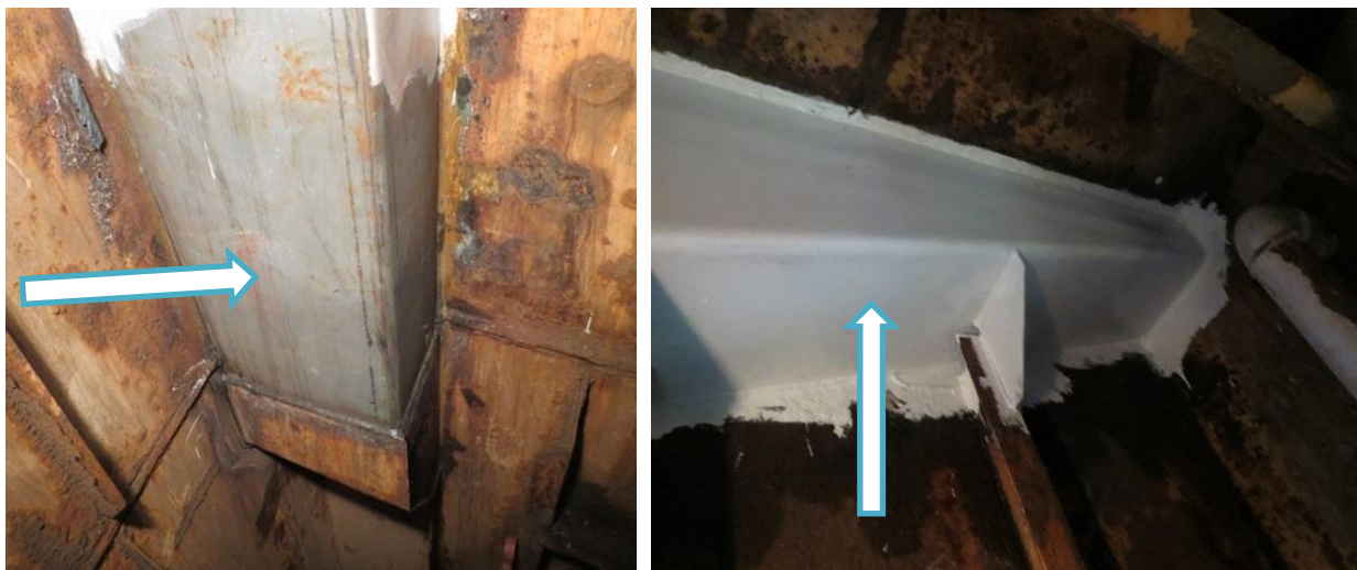
Photograph 8. Air conditioning ventilation trunk after the repair.
