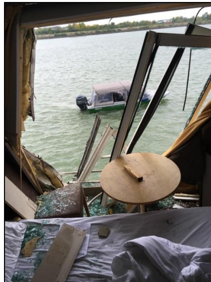
Figure 5.2 – Damages to Cabins
