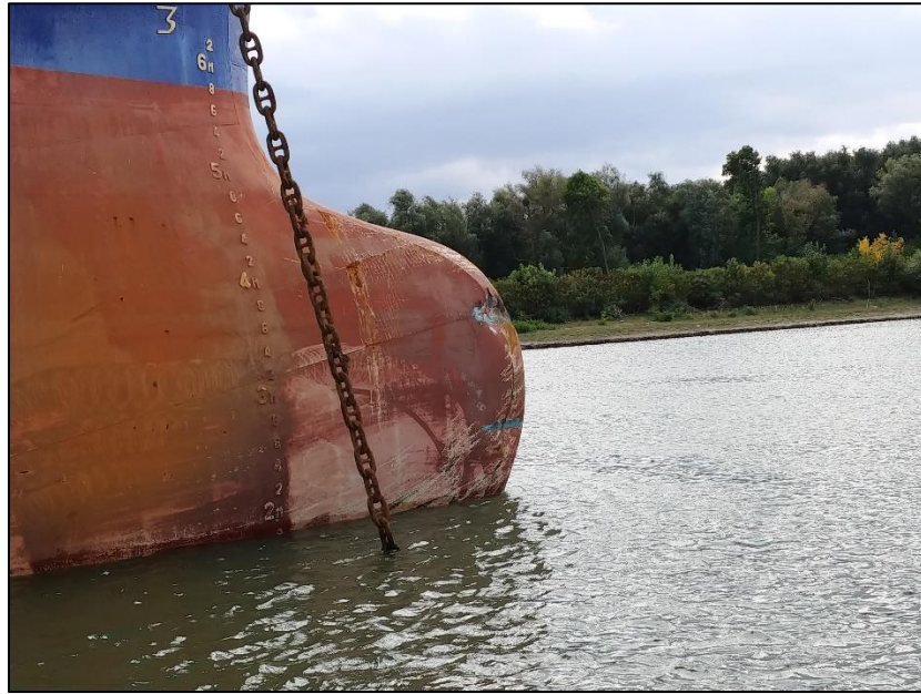
Figure 5.9 – Damages to bulbous bow
