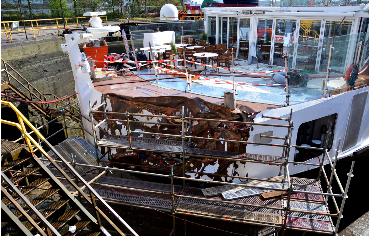
Figure 7: The damage to the bow of the Viking Idun, photographed in dry dock.
