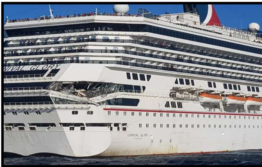
Figure 2: Affected area of Carnival Glory (deck 4 and deck 3 partially damaged)
