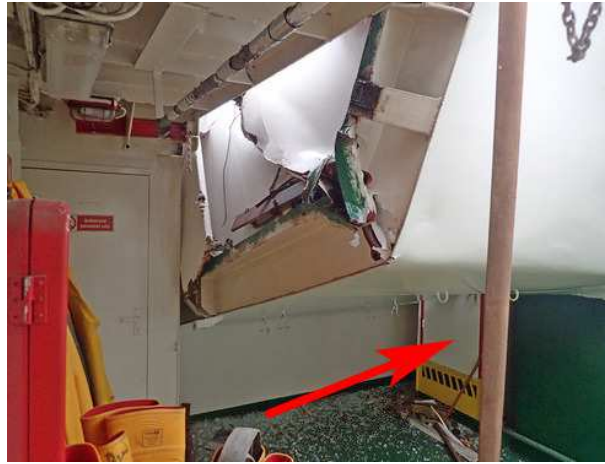
Access door to the accommodation. Source: gendarmerie
