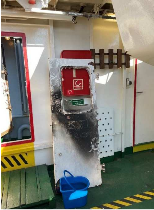
Starboard door of the bridge after removal and after cutting with a blowtorch. This door is also visible in the photos in 2.4
