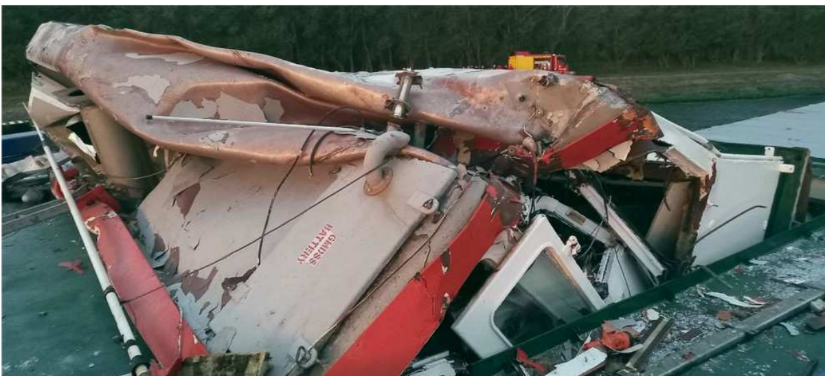
Tearing out and tilting of the wheelhouse, with roof compression - Source: VeriTech
