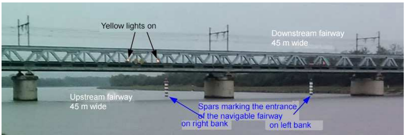
Railway bridge, downstream view
