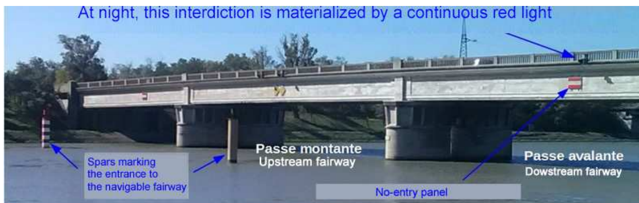
Road bridge, downstream view from left bank
