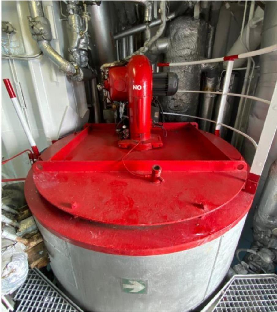
*Image 3 Boiler No.1 Currently Operating Onboard*
