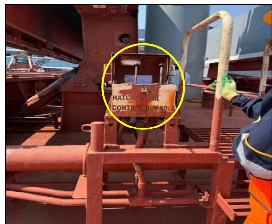
Figure 2: Cargo hold no. 2 hatch covers control station
